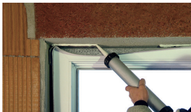
Installation example: ISO-TOP FLEX-ADHESIVE SP
