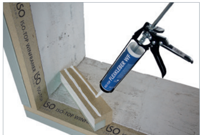
Installation example: ISO-TOP FLEX-ADHESIVE WF
