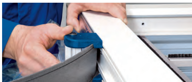
Installation example (CB): Fitting PVC windows
