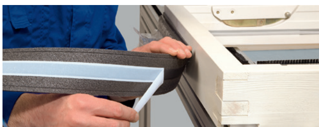
Installation example (1-BT): Fitting wooden windows
