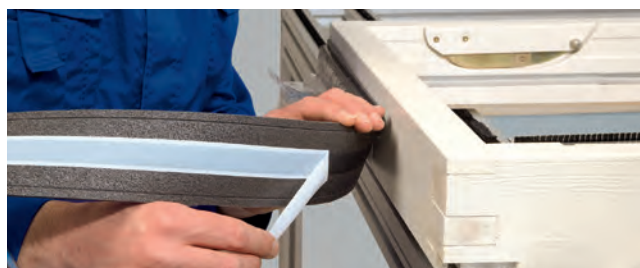
Installation example (1-BT): Fitting wooden windows
