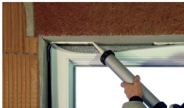
Installation example: ISO-TOP FLEX-ADHESIVE SP
