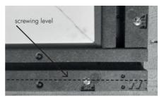
Only countersink the screw heads halfway into the material. If the screws cannot be fitted at the marked spacings, they should be distributed as follows:
