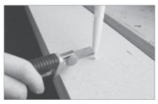
Adhesive is applied to the system profile as shown in the illustration below
