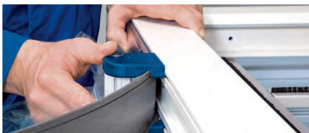
Installation example (CB): Fitting PVC windows
