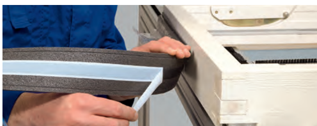
Installation example (1-BT): Fitting wooden windows
