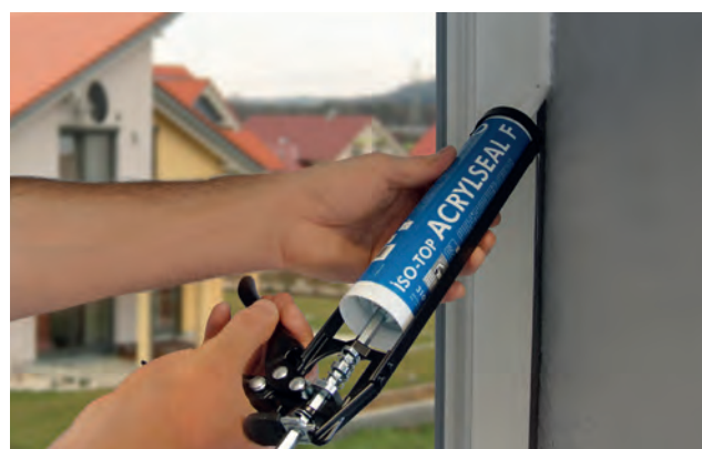
Installation example: ISO-TOP ACRYLSEAL F
