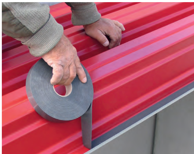
Installation example: ISO-ZELL FIX-TAPE
