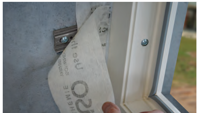
Installation example for ISO-CONNECT VARIO SD „PADS“
